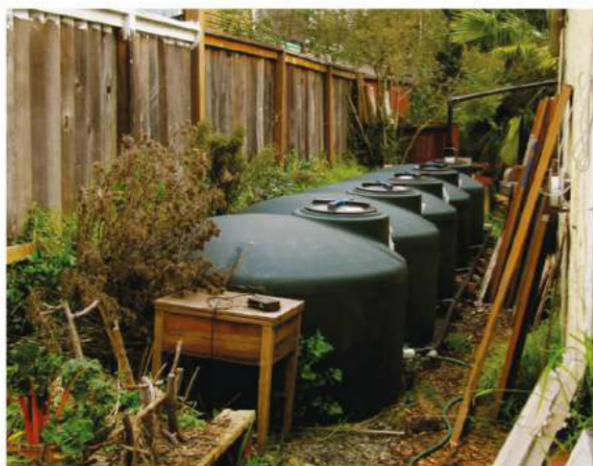
Top: Aquatic plants filter greywater in a repurposed bathtub. Bottom: Water tanks harvest rainwater on a useful scale.
